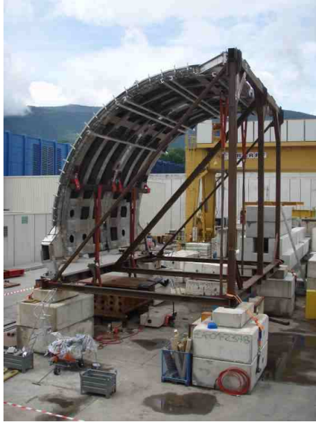
Figure 9.12: Setup used for the CalFrame load test.
